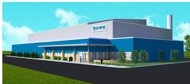
Construction of Production Facility to begin in 2019
